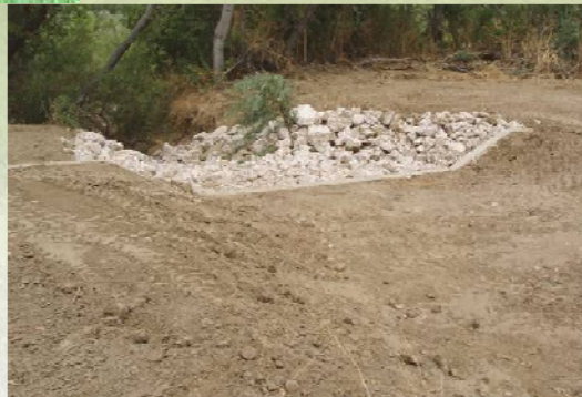
Concrete Grade Stabilization Structure w/ Rock Rip Rap
