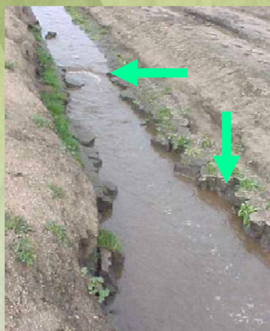
Bank erosion and channel downcutting in ditch
