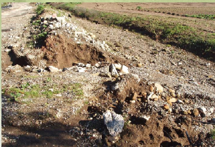
Soil erosion on unprotected ditchbank
