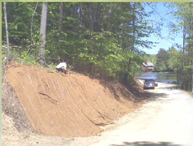
Cut bank stabilization – Erosion control blanket
