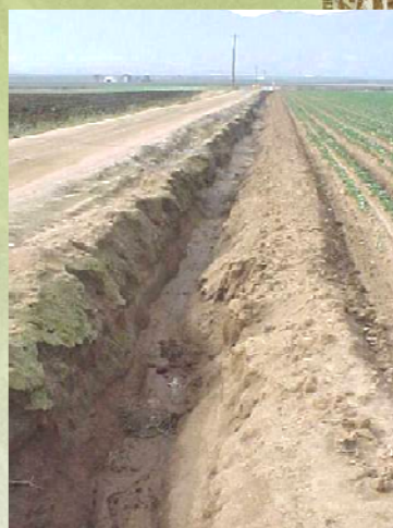
100+ cubic yards eroded per 1000 ft. of ditch
