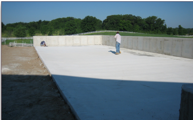
Figure 2. Concrete manure storage pad
