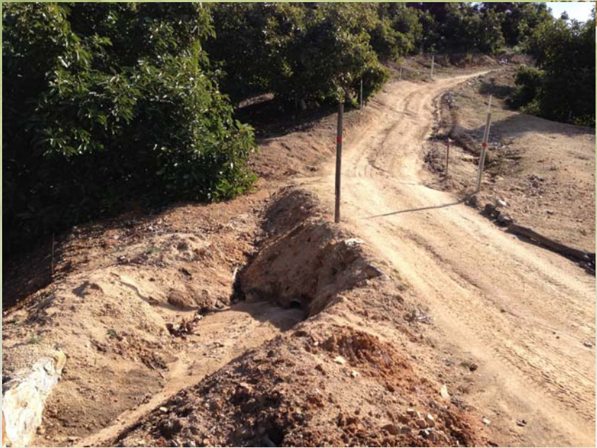
Rolling Dip with culvert
