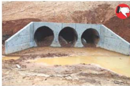
Poor seed and mulch application, slopes badly eroding. No rock apron or flow dissipater at culvert outlet. Culverts clogged with sediment and rock.
